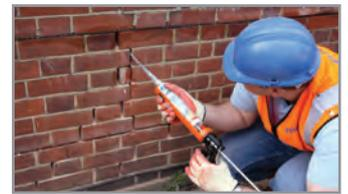
6. Re-point the mortar bed and make good the vertical crack with CrackBond TE3
