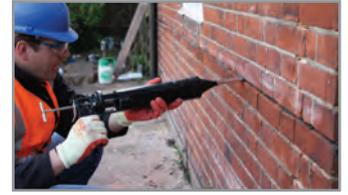
5. Insert a further bead of HeliBond over the exposed HeliBar, finishing 12mm from the face, and 'iron' firmly into the slot using the HeliBar Insertion Tool
