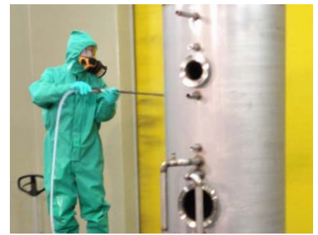
Photo: Application of Cleaner 401
